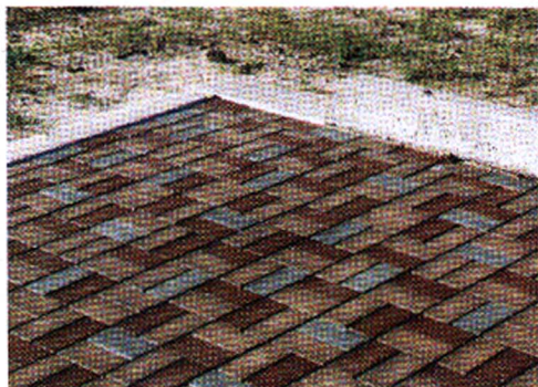
Permeable pavers can free up land used previously for retaining ponds.
